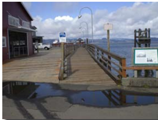
Public access constructed as a private/public partnership in conjunction with private development
