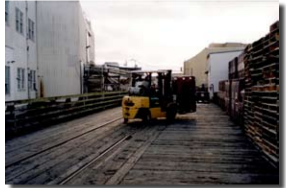
Astoria's "working waterfront" supports a mix of uses
