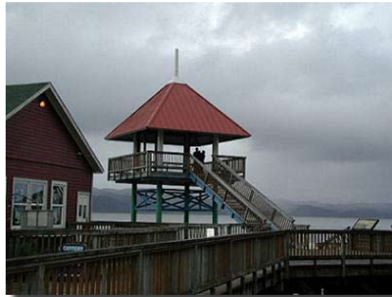
6th Street viewing platform
