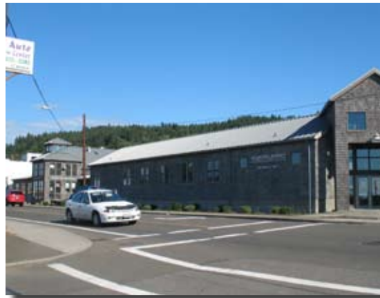
Create safe pedestrian crossings
