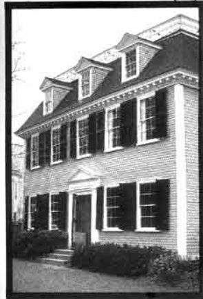
Henry Vassal House, Cambridge, Mass. (1746). Skived clapboard, 3 1/2-inch exposure.
