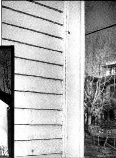
Silas Deane House, Wethersfield, Conn. (c. 1766). Skived clapboard, 3-inch exposure.
