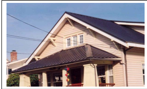
High profile metal seam roof
