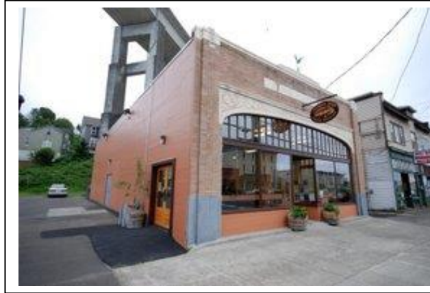
Figure 14.115-5: Non-Industrial Building, Flat Roof Behind Parapet Wall
