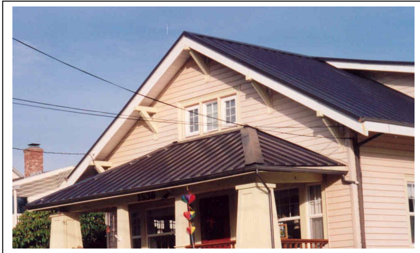
High profile metal seam roof
